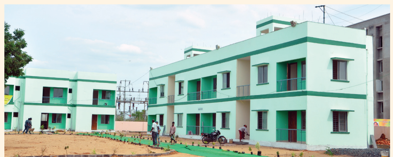
Demonstration Housing Project at SPSR Nellore, AP
